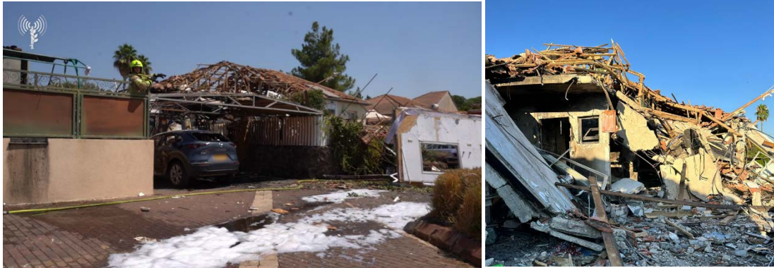
Buildings damaged in Katzrin (IDF spokesperson, August 21, 2024)
