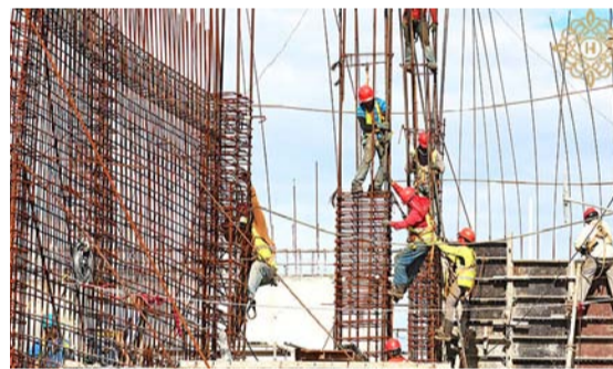
File photo depicts construction workers at a building site in Tehran.
