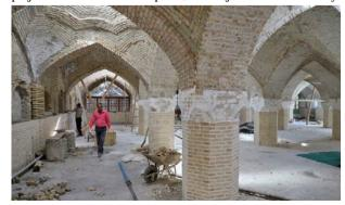
The project involves repairing the mosque's columns, walls, ceiling's insulation, arches, and gutters as well as replacing worn-out materials and lightening roofs, the official added
